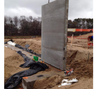
First wall up this week
