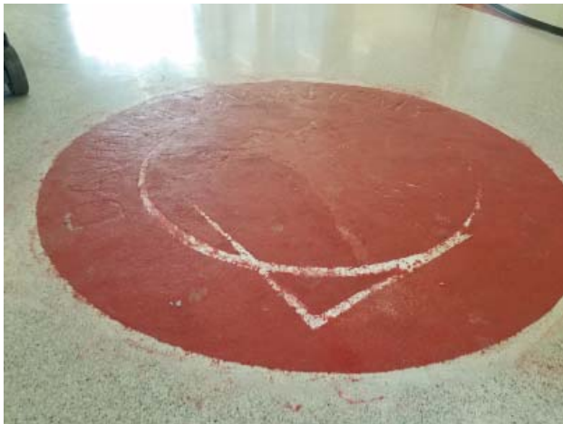
Terrazzo logo is poured as of 9/15/17 and soon will be grinded and polished
