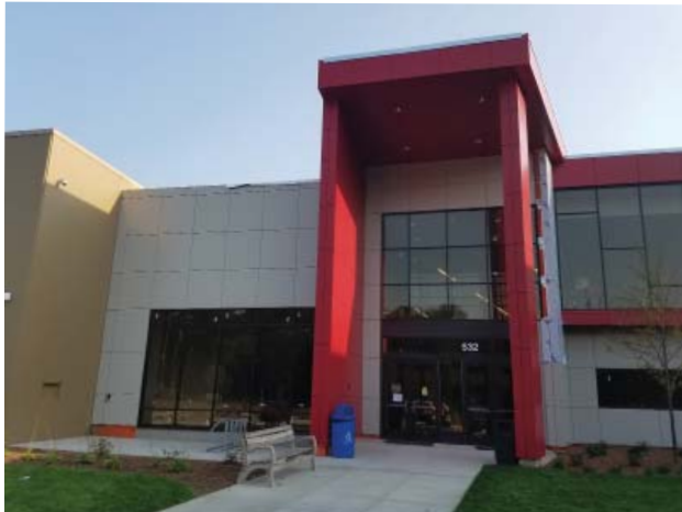
Exterior metal panel installed as of 9/15/17
