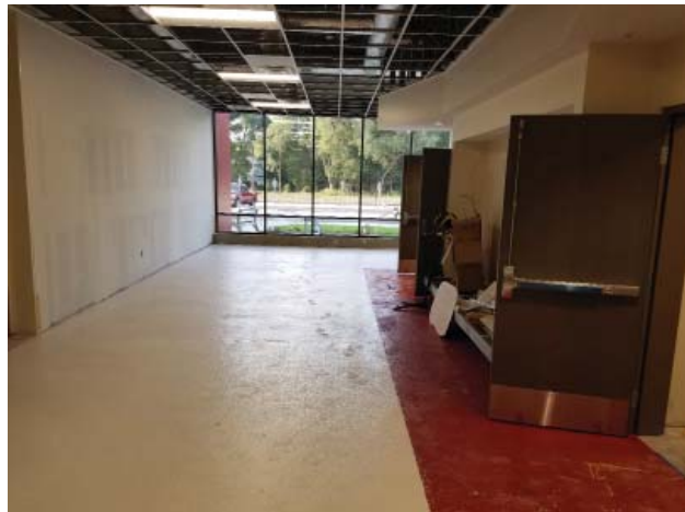
Breakout area west of the auditorium with terrazzo poured as of 9/15/17
